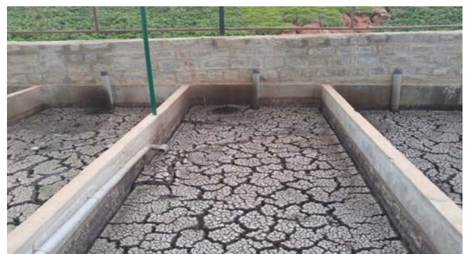
Figure 43: Sludge Drying Bed
