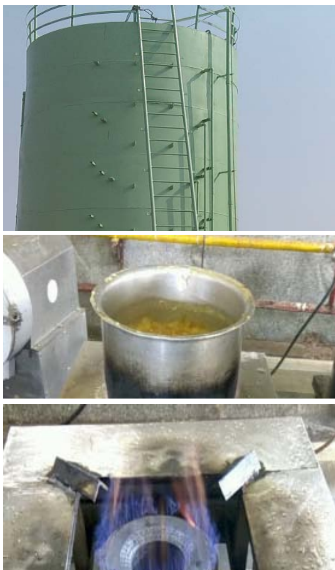
Figure 16: High Rate Biomethanation Plant at Toranagallu (Bellary), Karnataka
