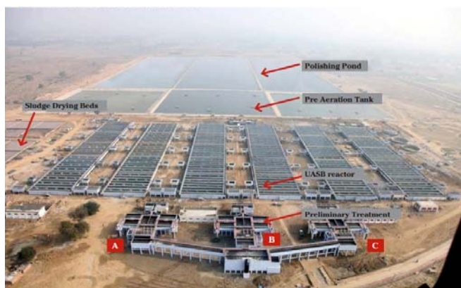
Figure 38: 345 MLD Lucknow UASB based STP along with Sludge Drying Bed
